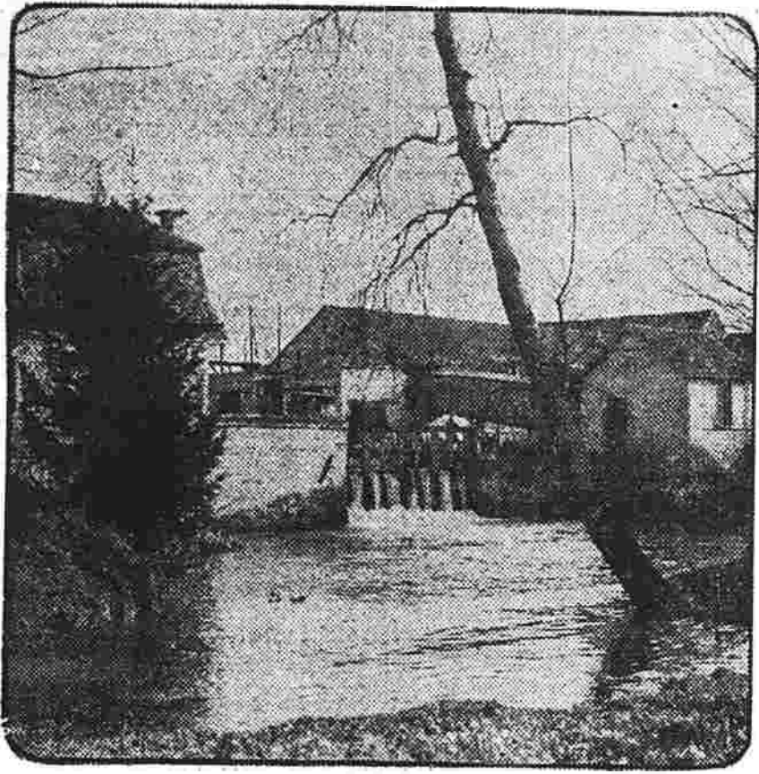
A reconstructed mill at St. Gilles, on the Vesle. Nine years ago this water was flowing red.
